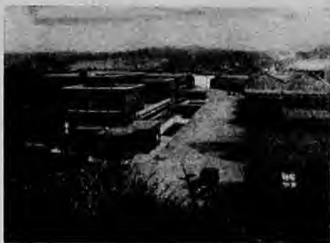
Above—The General Offices, 1936.
